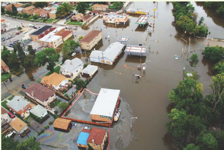
September 2008 flooding in communities along the Des Plaines River, southwest of Chicago. Metropolitan Water Reclamation District of Greater Chicago, ©MWRDGC2012-01.
